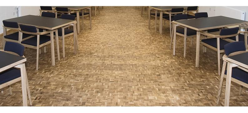
**HØRNING End Grain Mosaic** is made of small solid square blocks just like end grain flooring, which are cut opposite the annual year rings.
